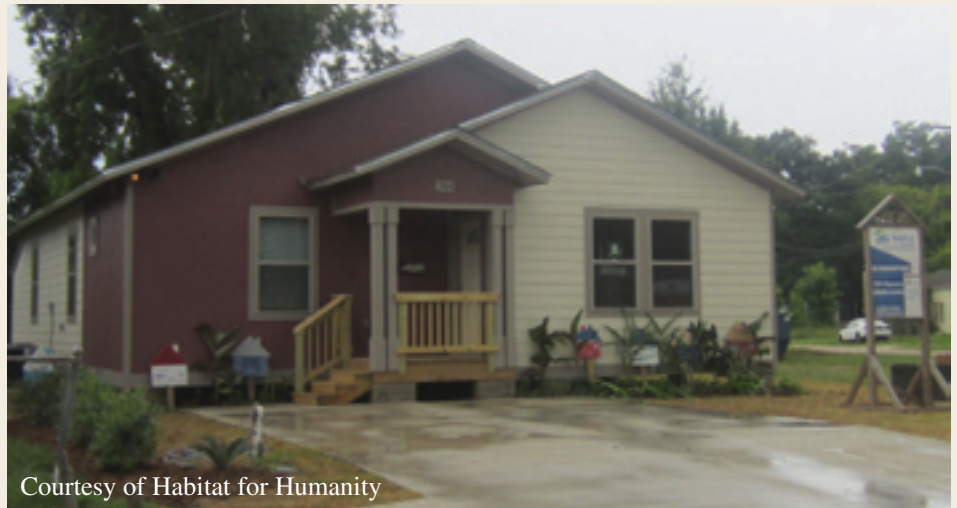
Courtesy of Habitat for Humanity
