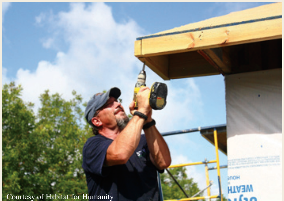
Courtesy of Habitat for Humanity
